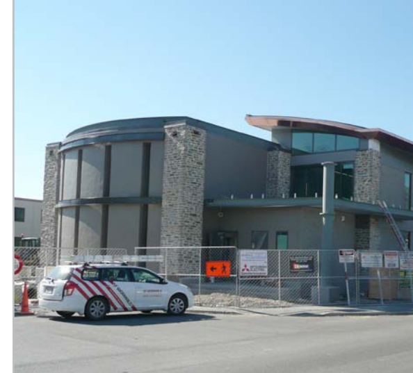
Construction at 190 Waenga Drive is underway
